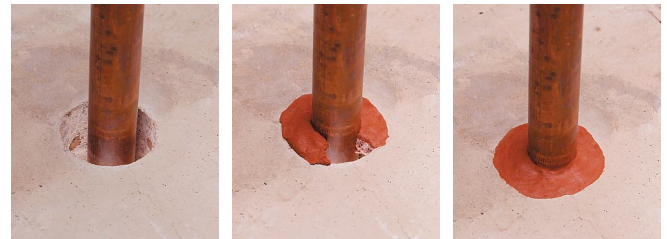
Through-penetration being firestopped.
