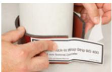
Wrap  $3M^{\text{TM}}$  Fire Barrier Tuck-In Wrap Strip around pipe, over floor opening, and adhere label to adjacent side of foam strip.
