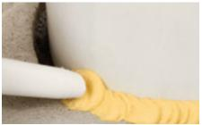
Follow wrap installation with layer of 3M™ Fire Barrier Sealant CP 25 WB+, IC 15 WB+, or 3000 WT to create seal that meets code, fire-rated to 3 hours.
