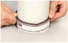
Gently slide wrap strip downward into concrete floor to fill gaps.
